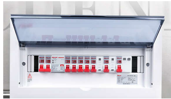
Step 2: Switch the input line to ON
